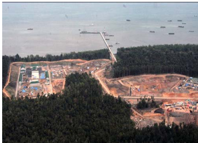
BP Shorbase Construction in Tanah Merah - Bintuni Bay
